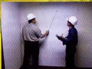
Checking hollowness of internal wall
