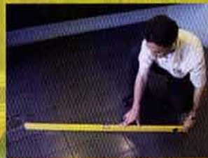
Checking fall of floor in wet areas
