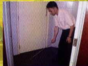
Checking hollowness of tiled floor
