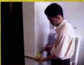
Checking squareness of internal wall
