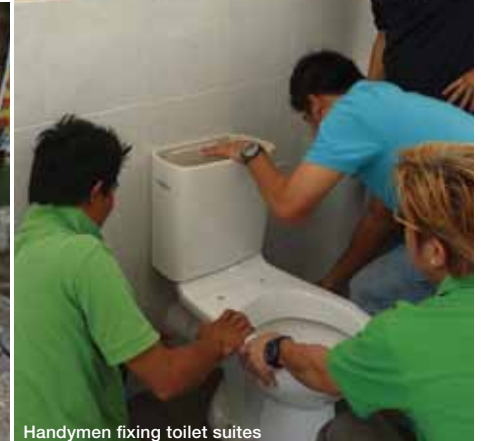
Handymen fixing toilet suites
