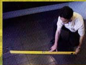
Checking fall of floor in wet areas
