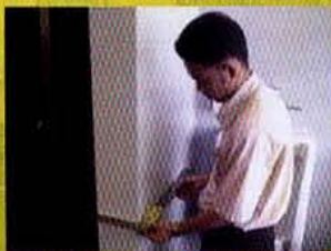
Checking squareness of internal wall
