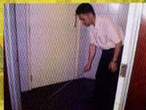
Checking hollowness of tiled floor
