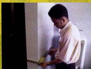
Checking squareness of internal wall
