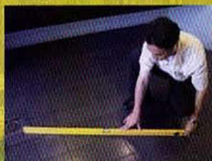
Checking fall of floor in wet areas
