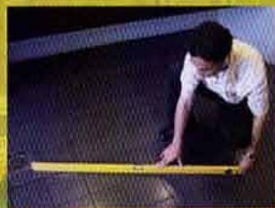
Checking fall of floor in wet areas
