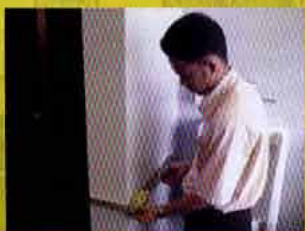
Checking squareness of internal wall
