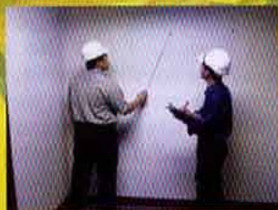
Checking hollowness of internal wall
