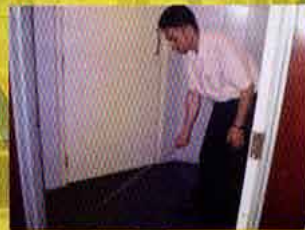
Checking hollowness of tiled floor
