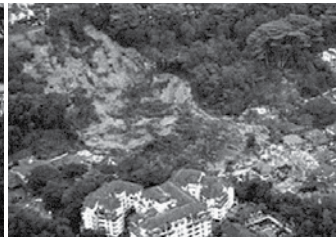
A view of a landslide in Kuala Lumpur, Malaysia, Saturday 6 December 2008. source: AP Photo/Royal Malaysian Police
