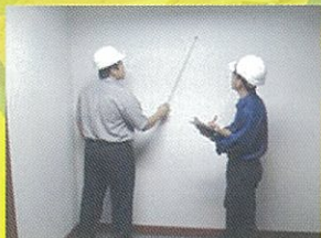
Checking hollowness of internal wall
