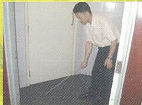
Checking hollowness of tiled floor
