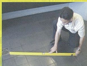
Checking fall of floor in wet areas
