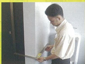
Checking squareness of internal wall
