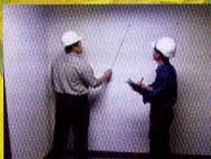
Checking hollowness of internal wall
