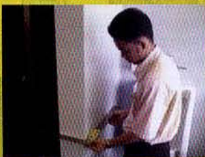
Checking squareness of internal wall
