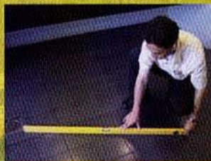
Checking fall of floor in wet areas
