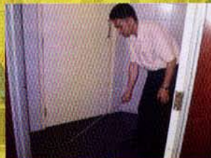
Checking hollowness of tiled floor
