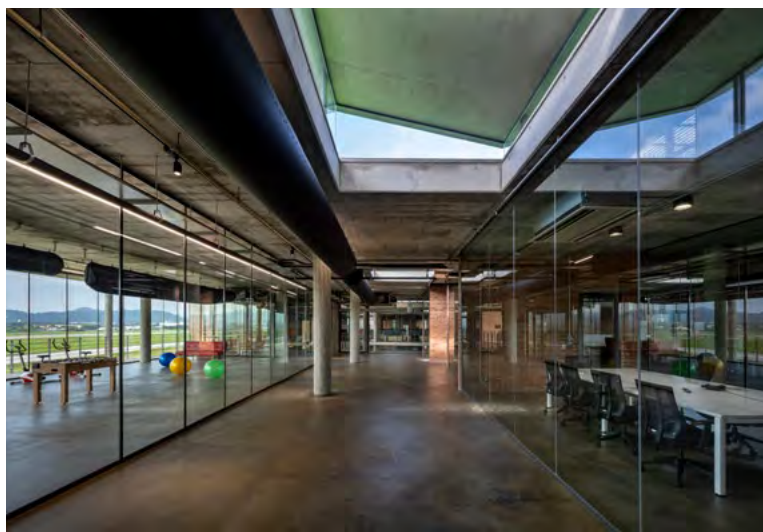
Roof lights at second floor provide diffused natural light across the office floor. Glazed meeting rooms allow views to the runway from deep within the building
