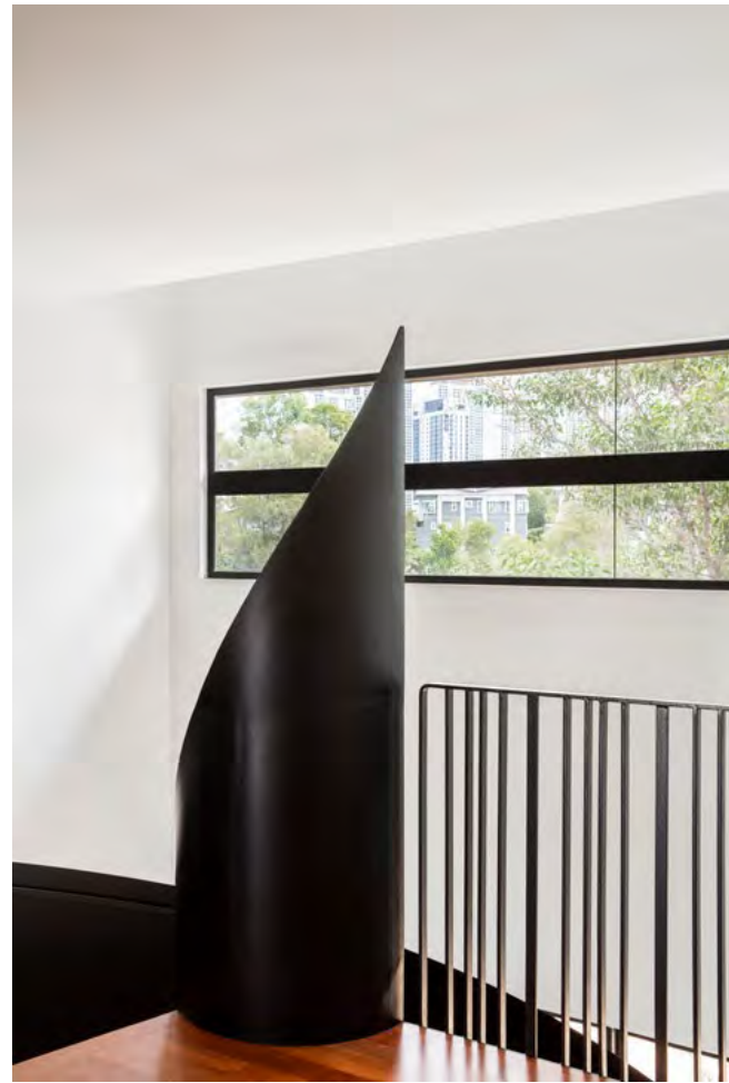
A dramatic solid curved plane of the stair's railing
