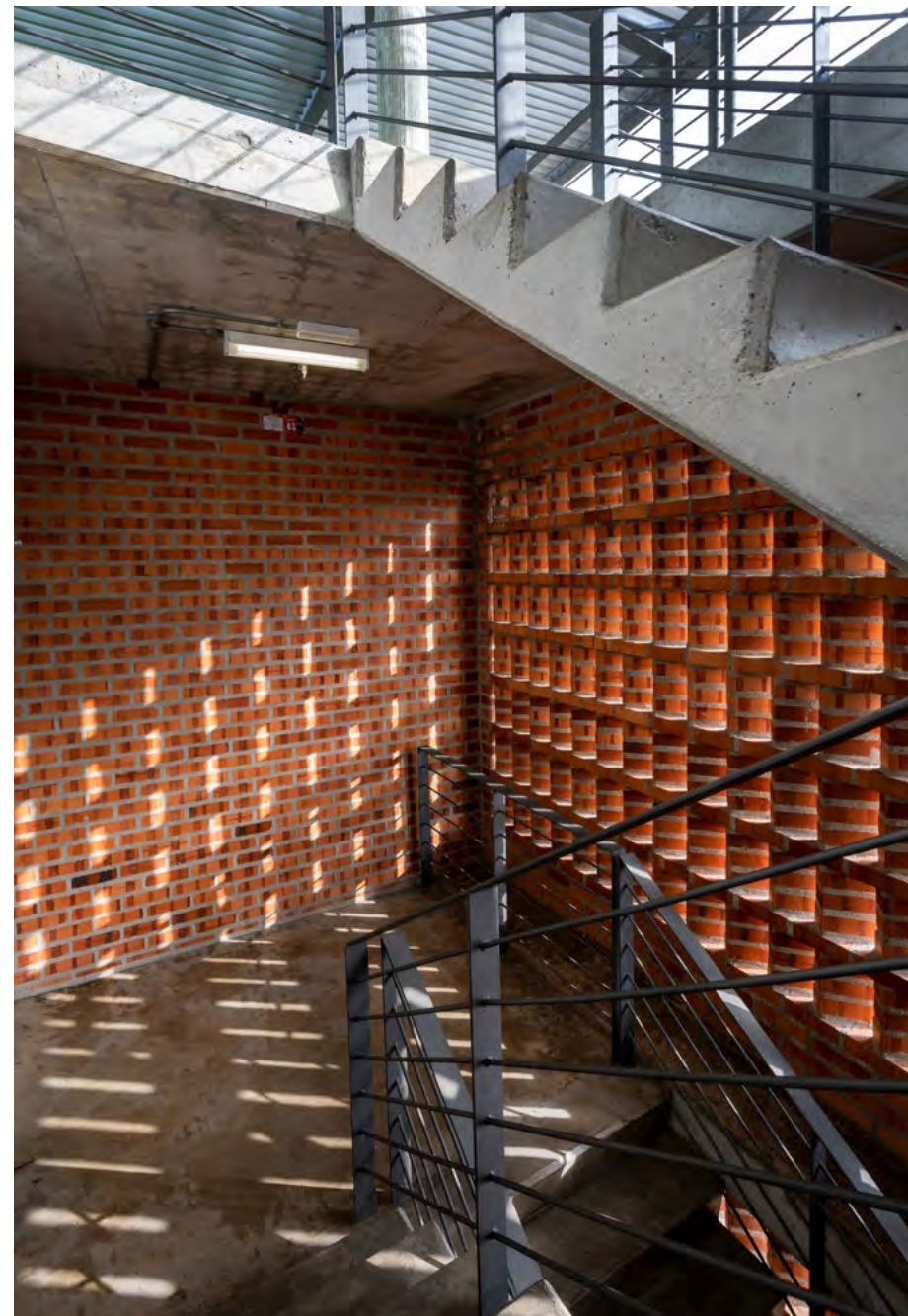
Perforated brick walls create magical lighting displays at production, staircases and WCs
