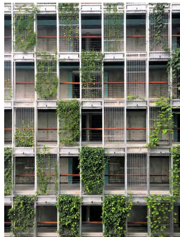
Green facade with automated irrigation system
