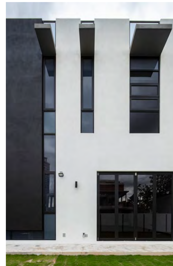
The northwest facade, facing the setting sun, was designed with minimal openings
