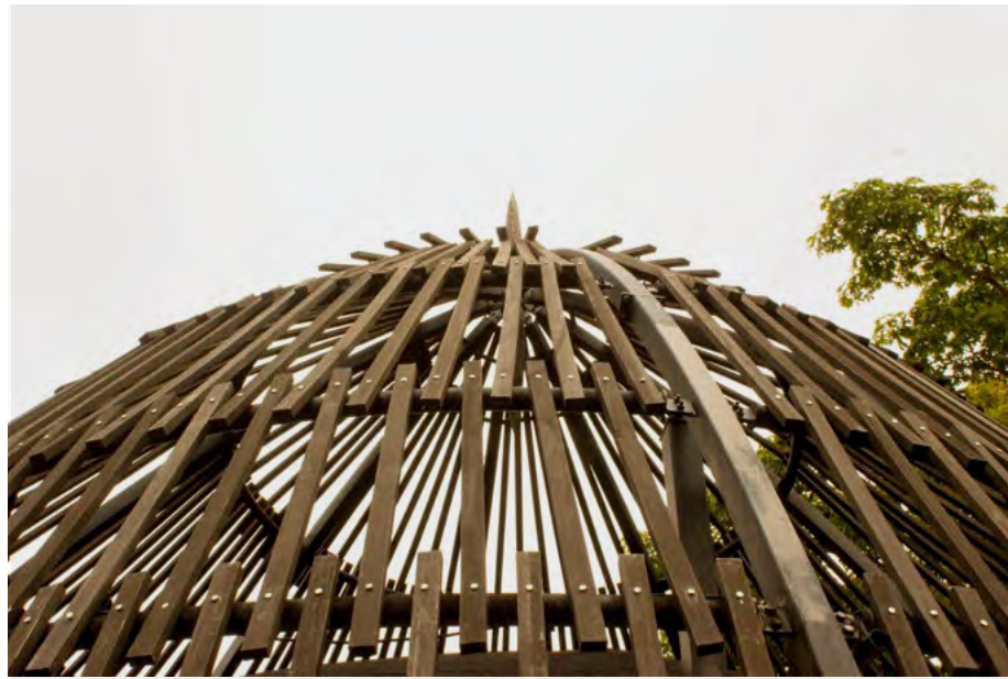
Curved laminated timber detail and connecting frame
