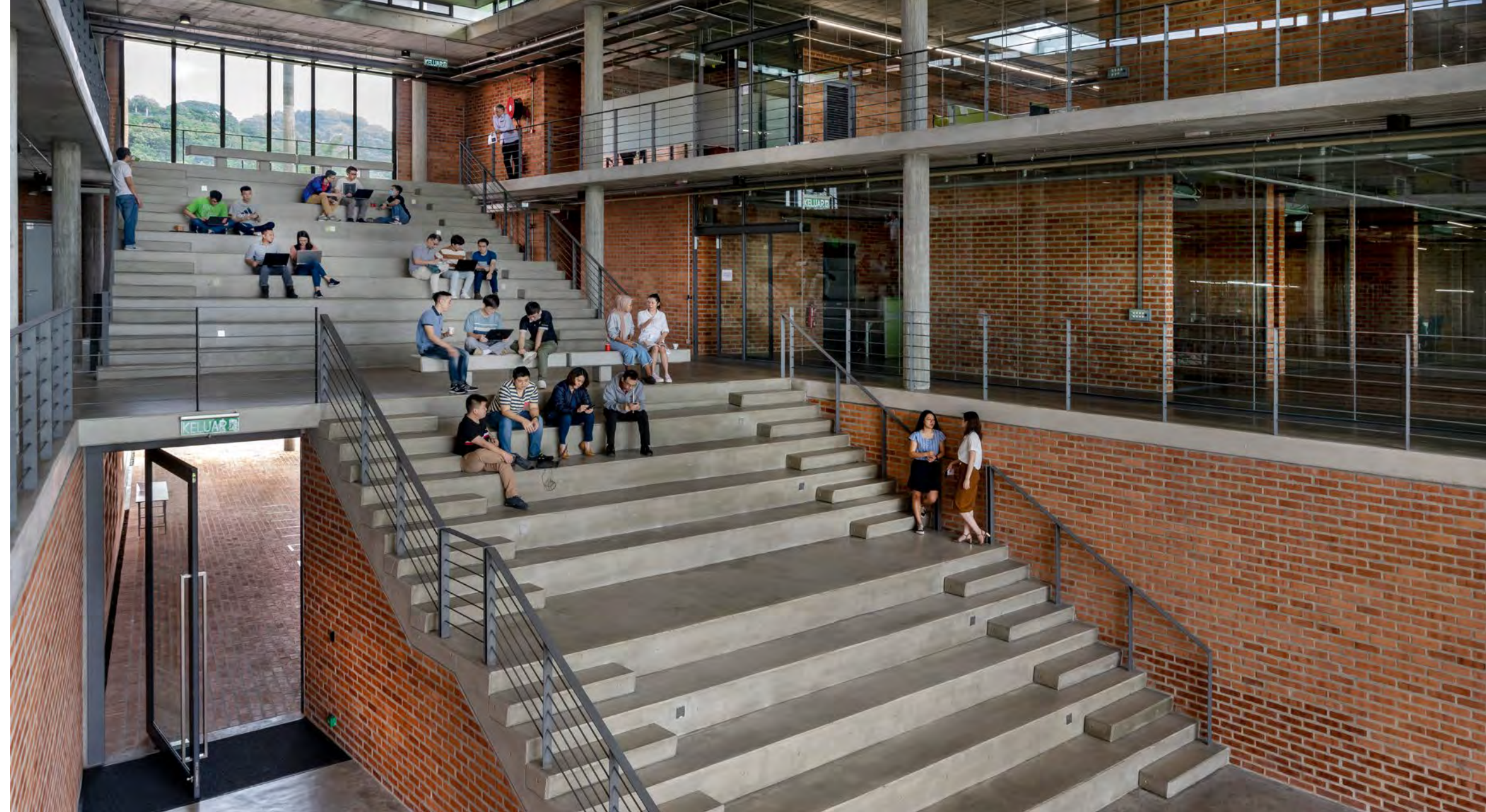
A large gathering space is created that connect all levels of the building. The atrium provides a flexible space for meetings, performances, theatre and dance
