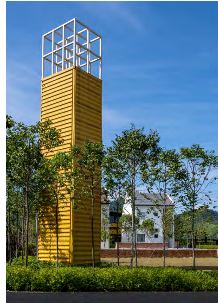
The beacon tower, made from a shipping container turned on its side
