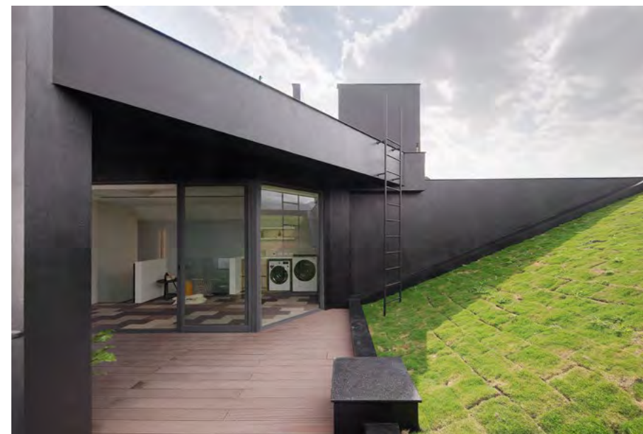
Green roof detail
