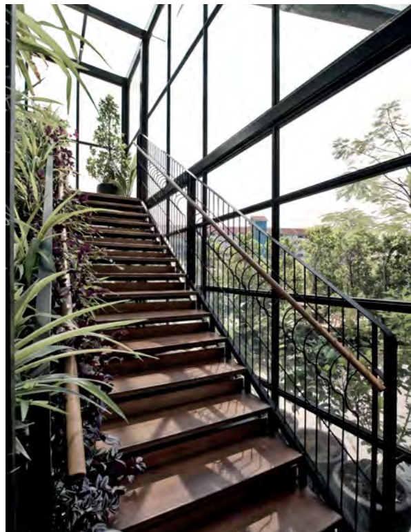
The new stairs leading up to mezzanine in the extended area
