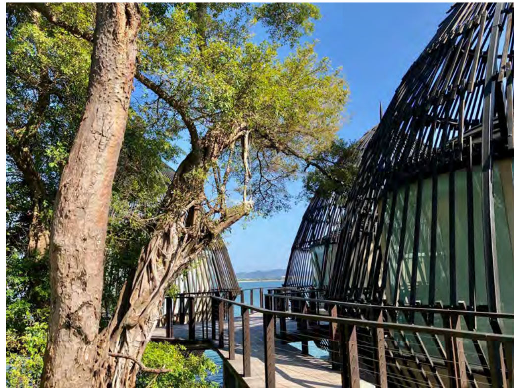
Spa bubu in site context of tropical trees
