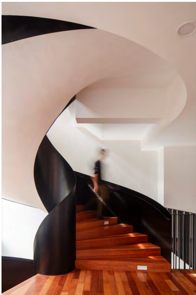
The spiral stairs with flat metal plate railing
