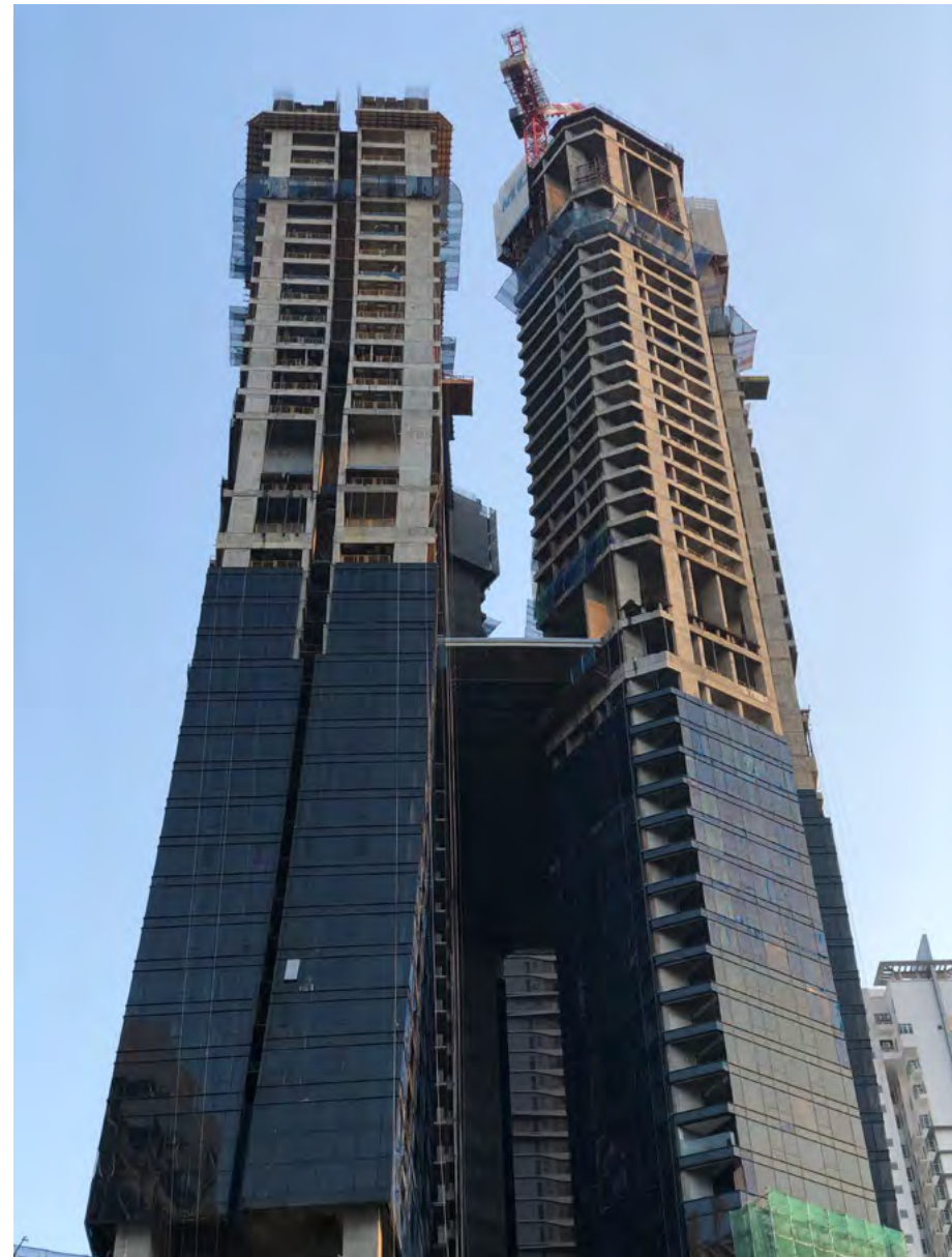
8 Conlay under construction
