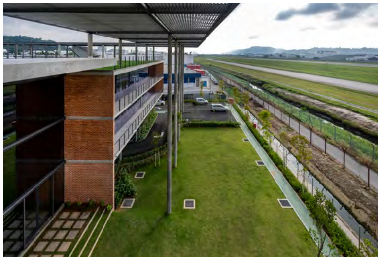
Runway views from shaded roof garden. The façade facing the runway is fully double-glazed and protected from solar gain by deep recesses and louvered canopy
