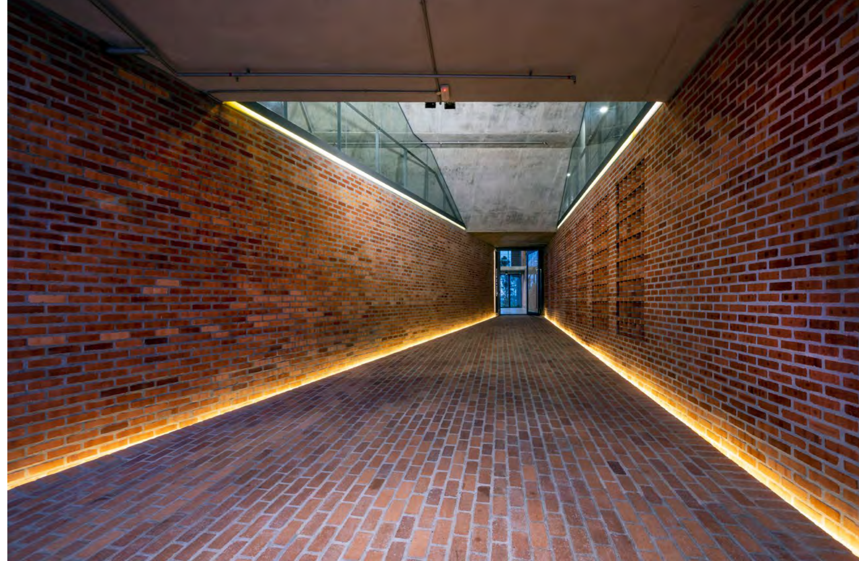
View of entrance tunnel. Walls, floor and ceiling all taper and converge to the main entrance door
