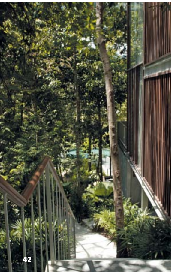
FROM LEFT: Facade exterior; Entrance bridge; External open deck
