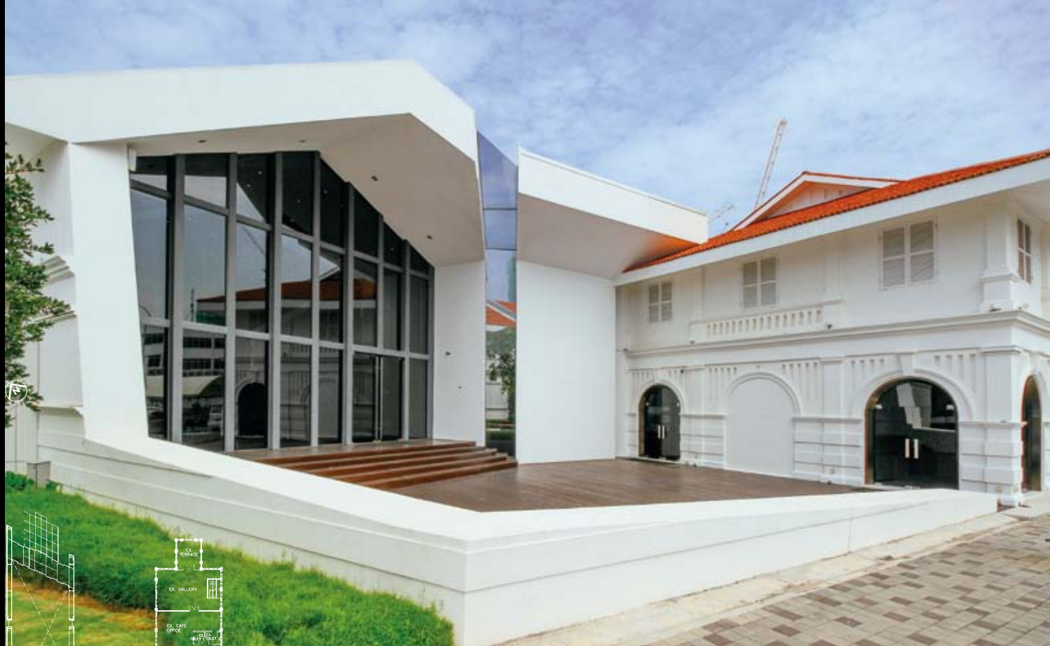
Intersection where the new building meets the existing building
