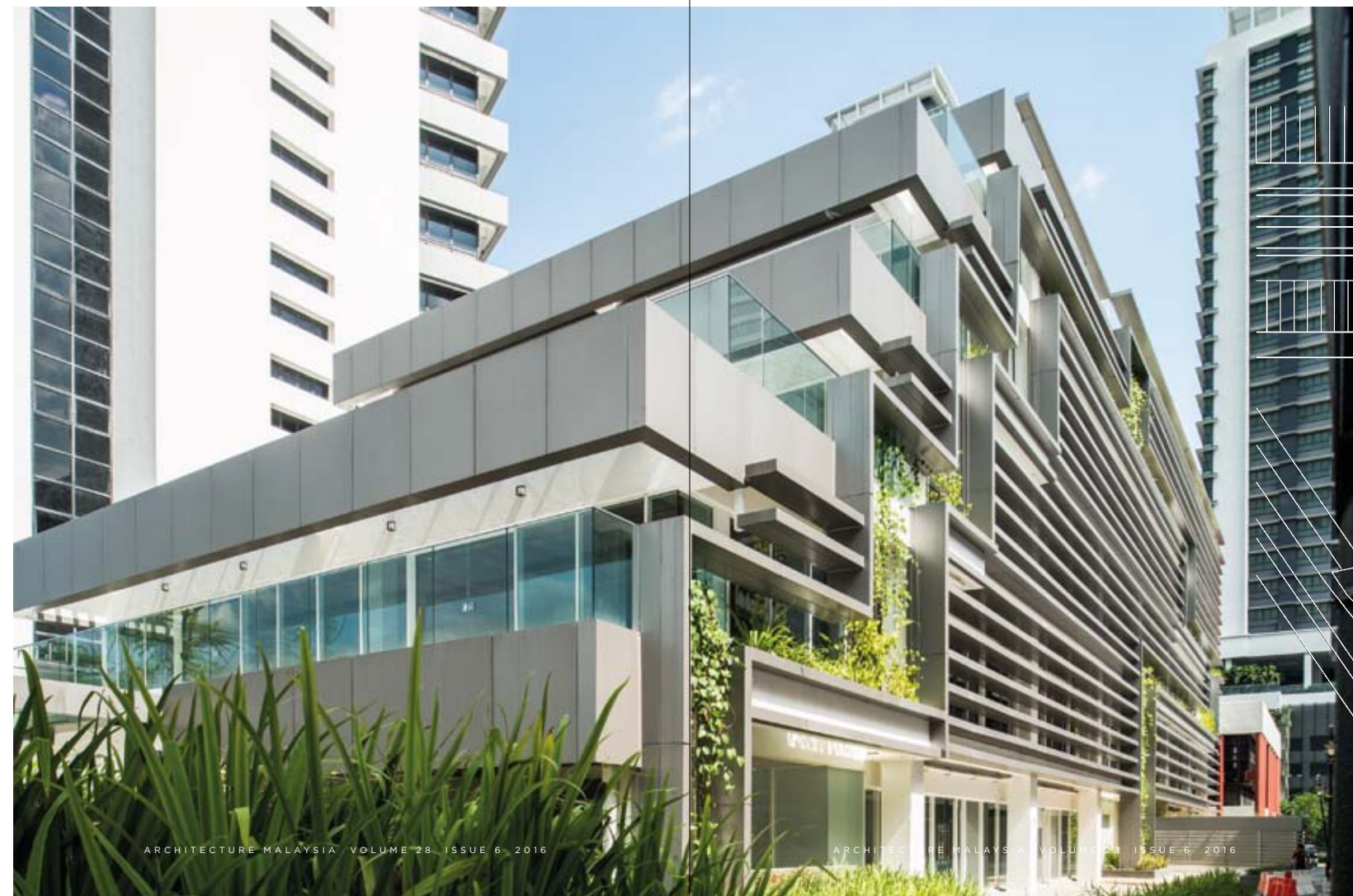
The stepped facade of the Annexe building
