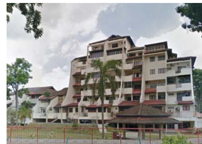
Trellis Apartments is an example of bioclimatic-based approach and pitched roof to establish a link to the locality
