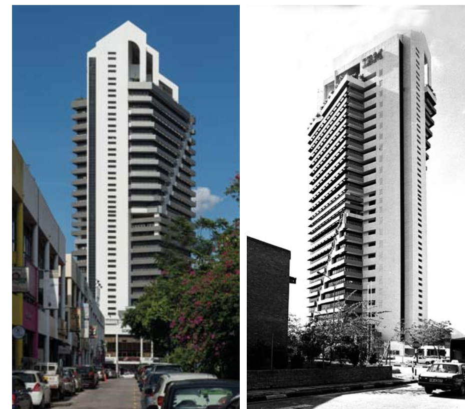
FROM LEFT: The subtly revamped and refreshed Plaza VADS; Archive photo of the former IBM Plaza
