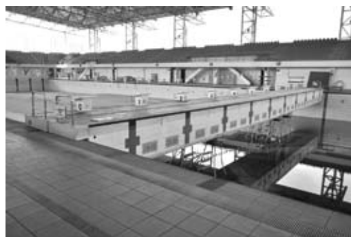
The existing Aquatic Centre before refurbishment works
