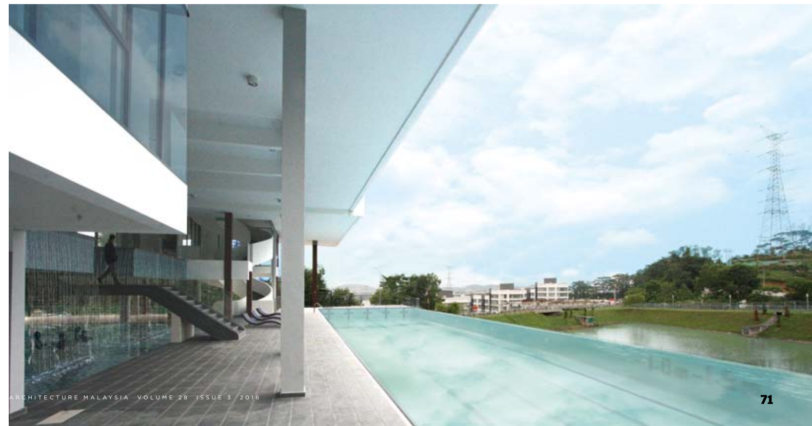
View towards the retention pond's community park, which has been integrated as part of the club
