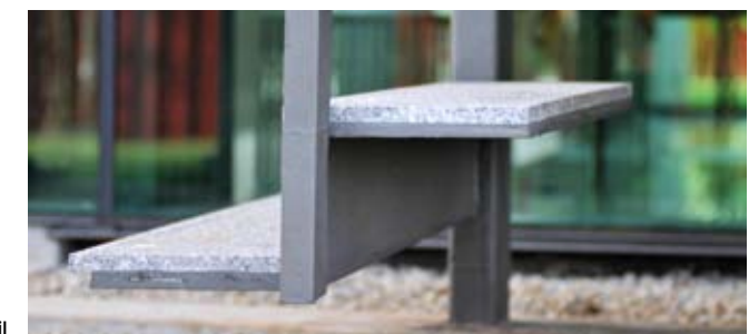
Hanging Z profile – staircase tread detail
