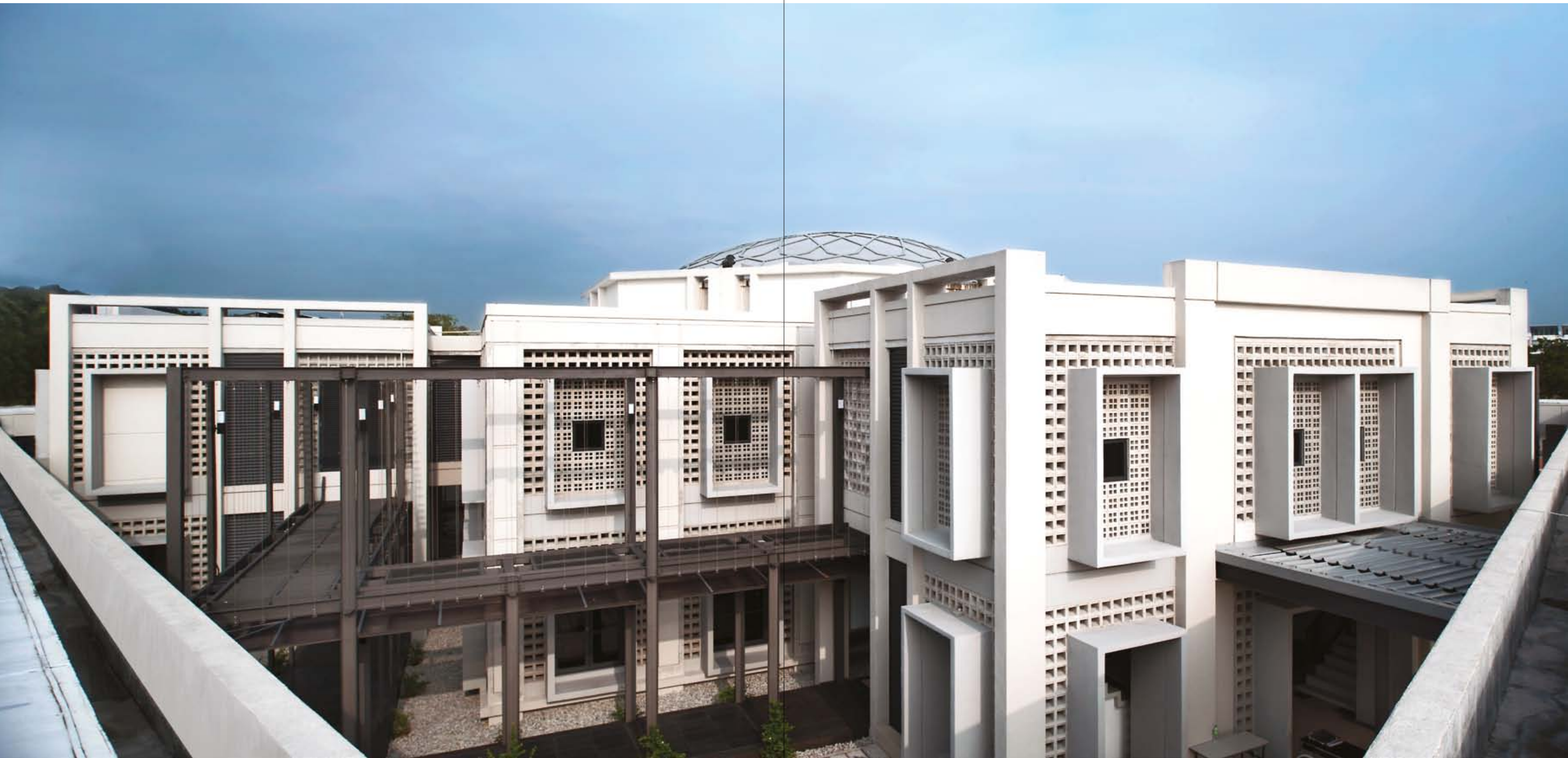
Elevation perspective that highlights the perforated skins that aid cross-ventilation and natural lighting
