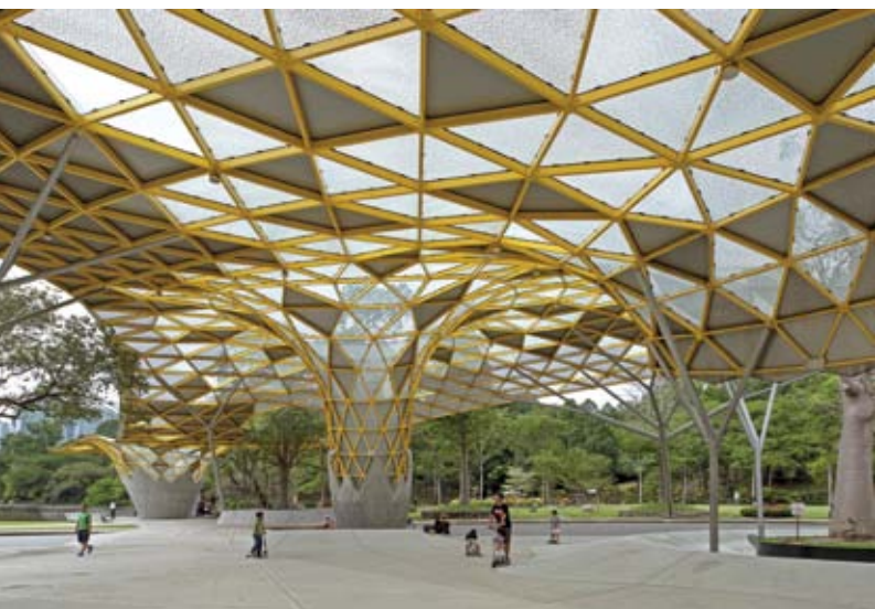
ABOVE: The Perdana Canopy is designed with consideration of the surrounding context, achieved subtly by emulating the organic fluid lines of the surrounding nature; RIGHT PAGE: The roof offers excellent shading device for any programmes
