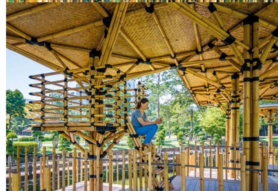
Bamboo baskets called 'tree-houses' add another dimension of space to the pavilion
