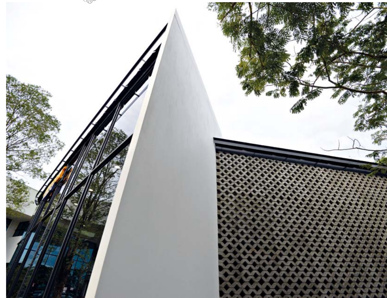
Three different wall treatments on the gym at a glance, varying from full-height glass panels, concrete to perforated grasscrete screens
