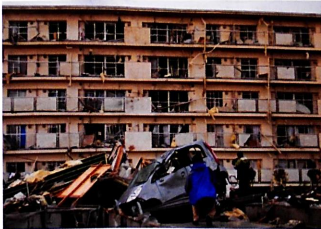
Photo 1 Example of damage caused by tornado (Tsukuba in 2012)
