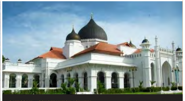
CATEGORY 7: CONSERVATION (SILVER) RESTORATION FOR COPPER DOME, ROOF & ASSOCIATED WORKS FOR MASJID KAPITAN KELING Arkitek Urbanisma Sdn Bhd
